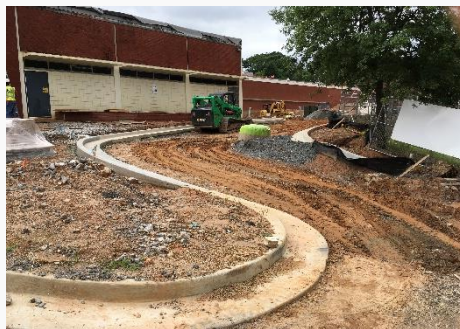
Curb and Gutter to Service Entrance
