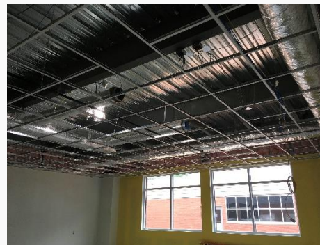
Ceiling Grid in Lower Level of Addition Building
