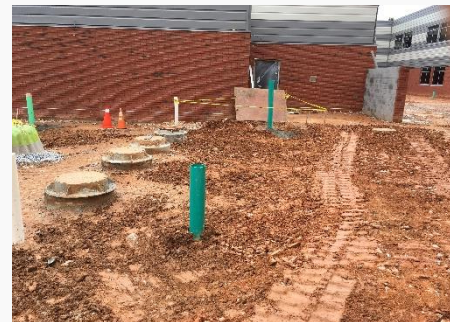
Manhole Covers to Finished Grade
