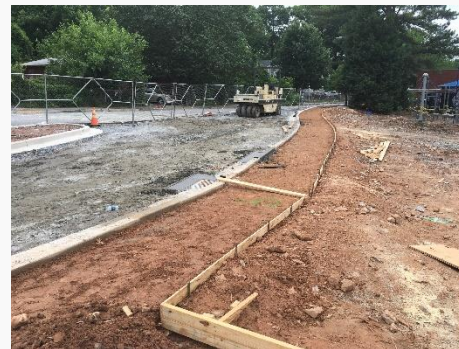
Prep. Framework for Sidewalk at Bus Loop
