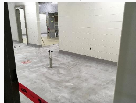
Preparation of Kitchen Service Area for Epoxy Flooring
